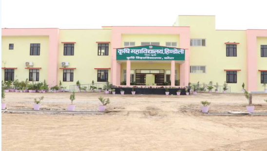
Construction of CoA, Hindoli completed
