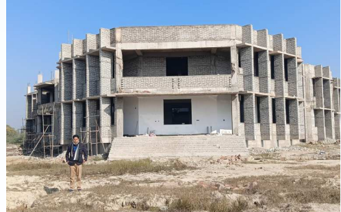
Construction of CoA, Kota in progress
